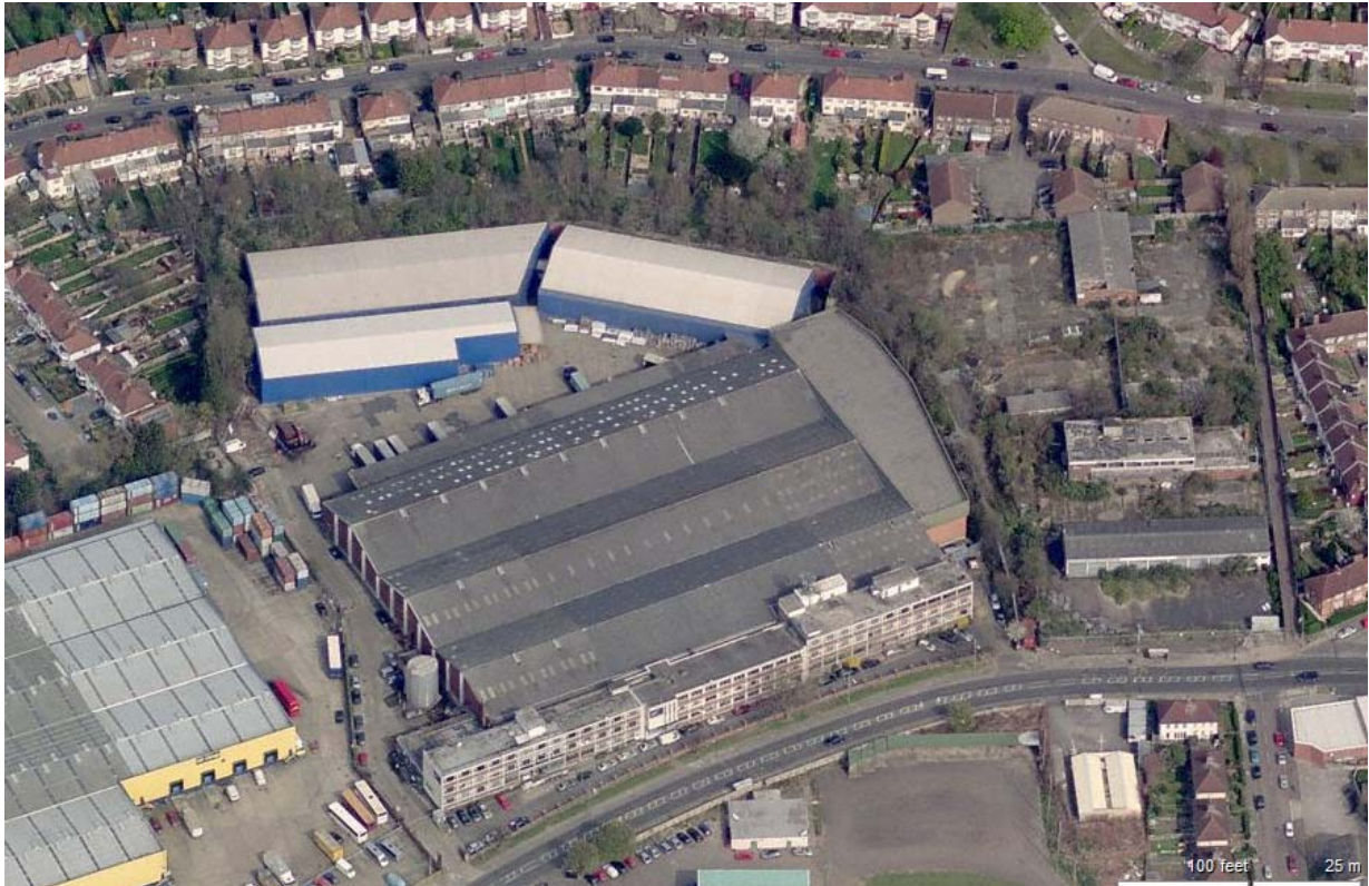
Figure 2: Aerial Photo of Previous Site Layout
